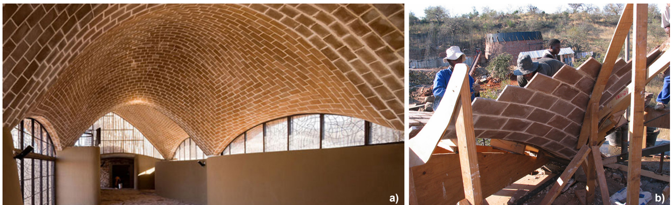
Figure 1. Mapungubwe National Park Interpretive Centre, Peter Rich Architects, (2008), a) interior view, b) under construction (Photo: James Bellamy).
