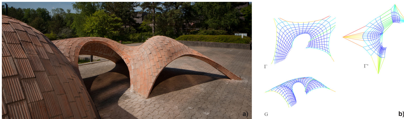
Figure 2. First free-form tile vault. BRG, ETH Zurich, 2011, a) finished vault (Photo: Klemen Breifuss), b) form diagram ( \Gamma ), force diagram ( \Gamma^* ) and 3D thrust network (G) (RhinoVault).
